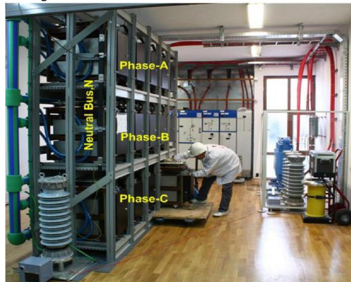
*Figure 3.1: Designed and implemented 3-phase, 12kV,  $\pm 12$  MVar, Y-connected 11-level CMC module*
